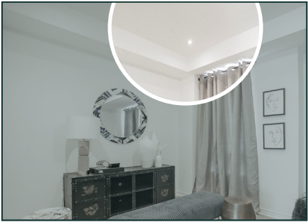
Smooth ceiling throughout (exluding basement)
