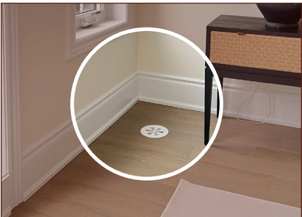
7-1/4" baseboards and 2-3/4" casing throughout
