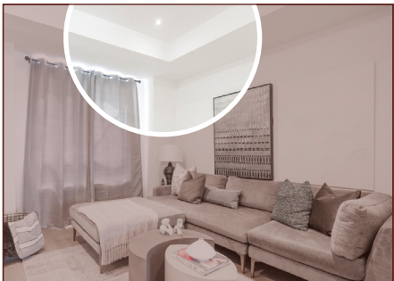
Coffered ceiling on second floor
